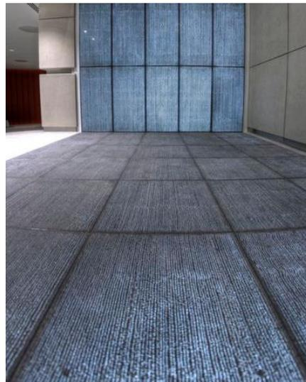
Figure 12 the first time to use transparent concrete in flooring in London & Oriental's London offices – features
