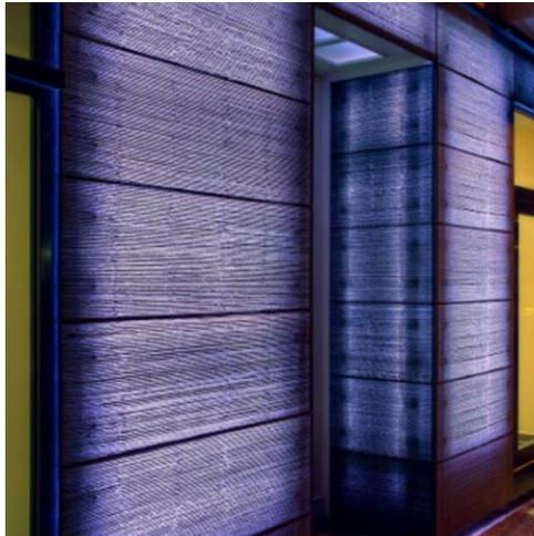
Figure 9 transparent concrete panels uses in wall cladding
